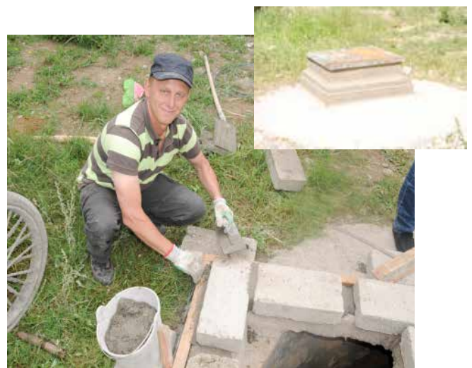
Andreas Schulz raising the level of the water collector in Dawu
